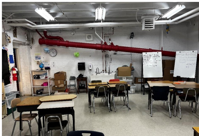
Existing Classroom Conditions
